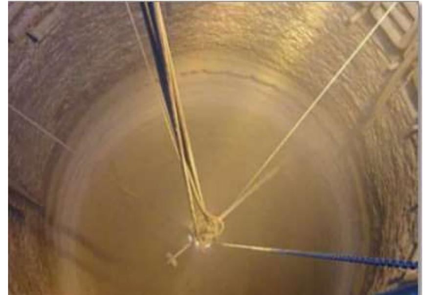
Device for the application of the inner coating of blast furnaces
